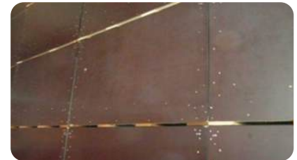
The difference creates a gap between the layers of the box, allowing the air that dried the product to escape.
